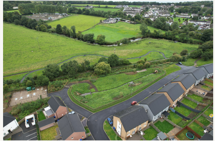
Aerial view of one of the SuDS basins, showing landscaping and the Six Mile Water
